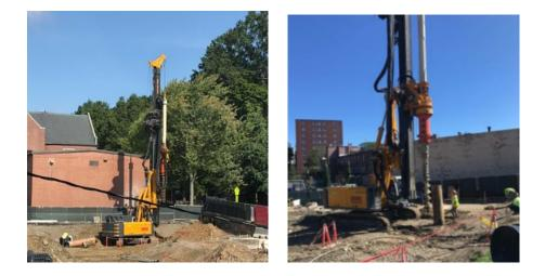
Shotcrete in preparation for soil nailing – 1<sup>st</sup> installation at NW corner
