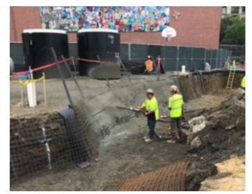
During construction unforeseen issues come up on the Project Site, the project team must make adjustments on and around the site to keep conditions safe for everyone. Recently we encountered a situation with heavy rain that washed out soil that had recently been excavated in preparation for the shotcrete and soil nailing operation. The construction team made the decision to close the walkway at the corner of the existing gym until an assessment and corrective work could be made at this location.
